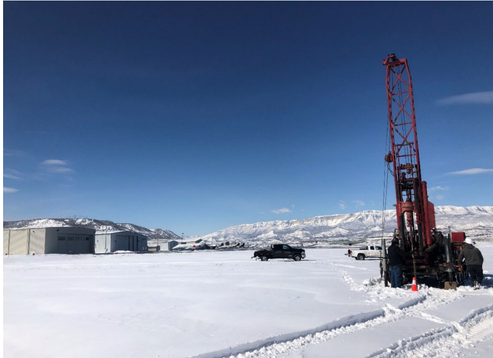
Figure 2. - Drilling boring B-1 looking west
