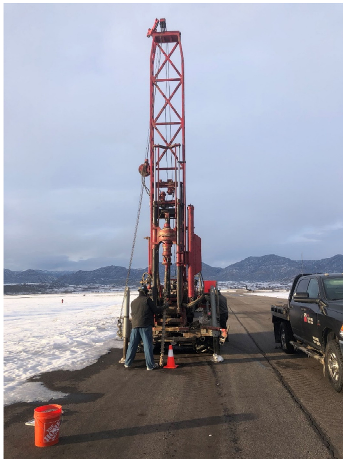
Figure 3 – Drilling boring B-3 at east edge Taxiway B4 looking north
