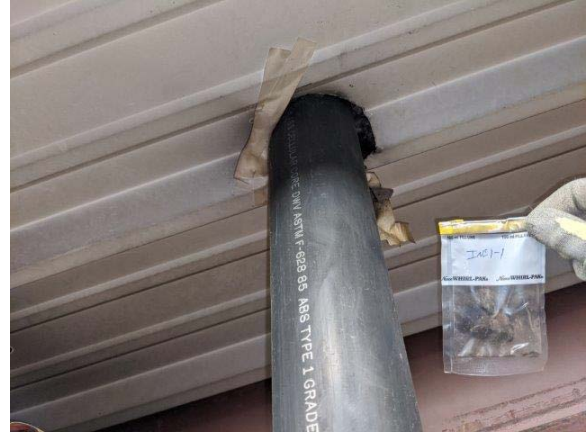
Sample: INS1-1 - Insulation, fiberglass Result: Non-Detect
