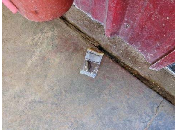
Sample: EJ1-1 - Expansion joint material Result: Non-Detect
