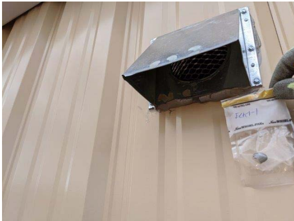
Sample: ECK1-1 - Exterior caulk, silver Result: Non-Detect
