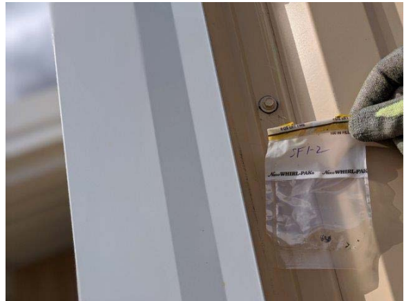
Sample: SF1-2 - Screw flashing Result: Non-Detect
