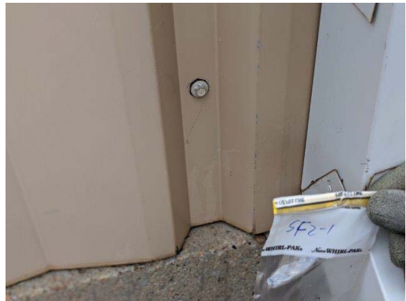
Sample: SF2-1 - Screw flashing Result: Non-Detect
