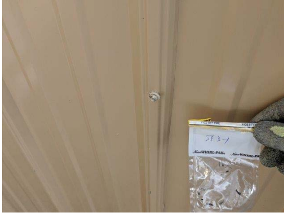
Sample: SF3-1 - Screw flashing Result: Non-Detect
