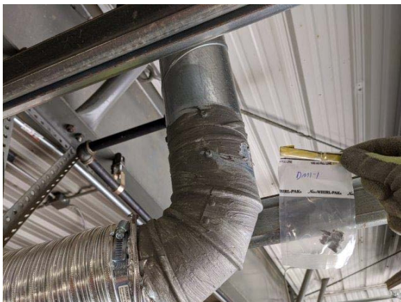
Sample: DM1-1 - Duct mastic, gray Result: Non-Detect
