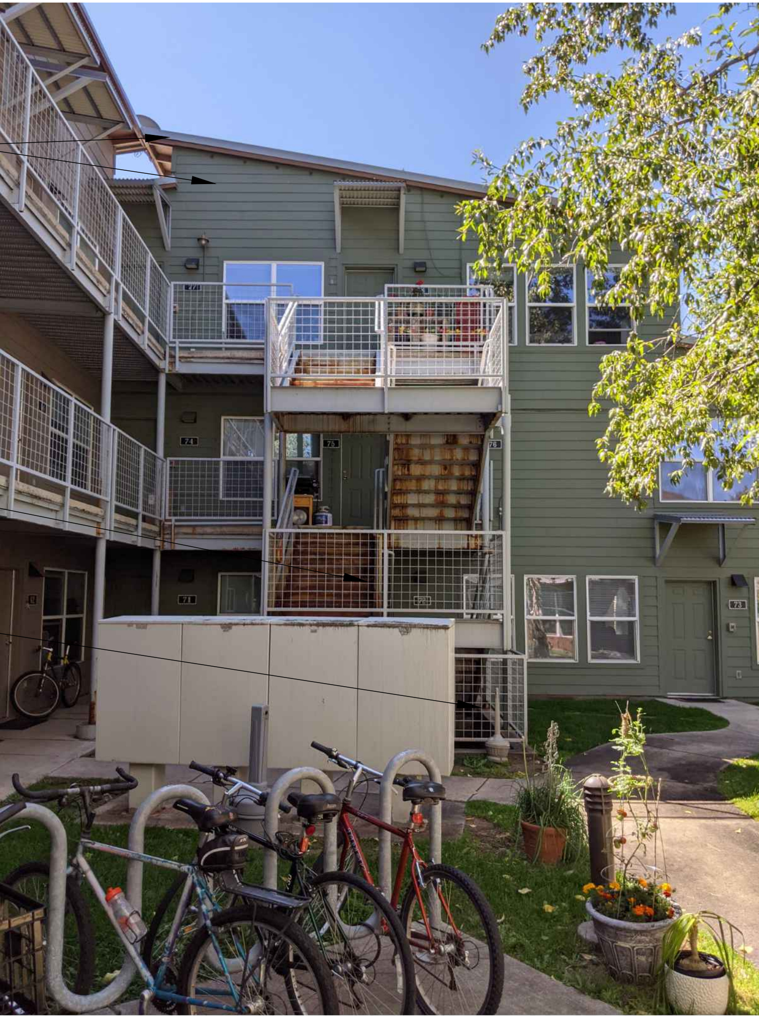
STAIR 70 (PHASE 4) EXISTING/DEMOLITION PHOTO 4 D1.4 NOT TO SCALE
