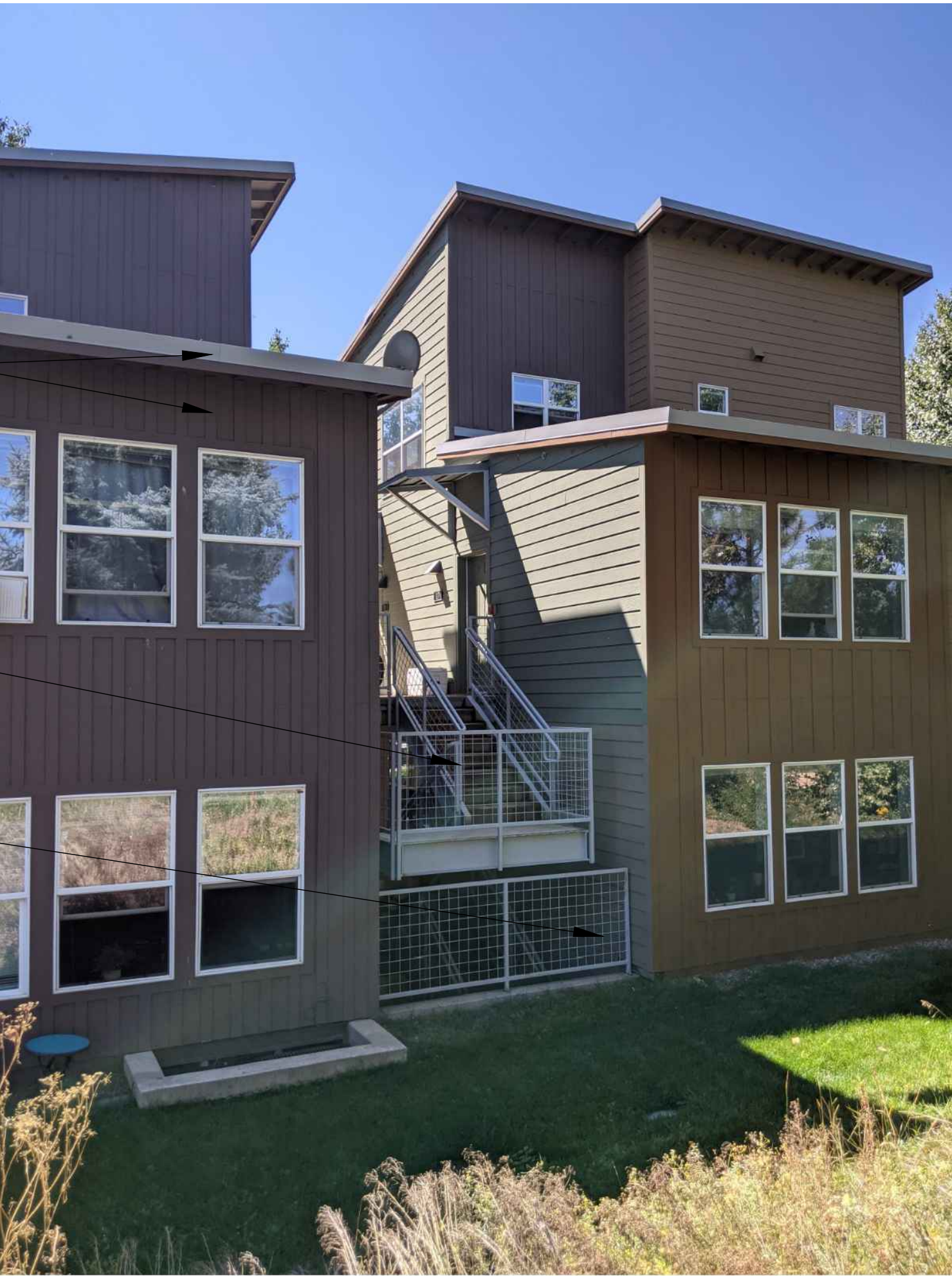
STAIR 20 (PHASE 2) EXISTING/DEMOLITION PHOTO 2 D1.4 NOT TO SCALE
