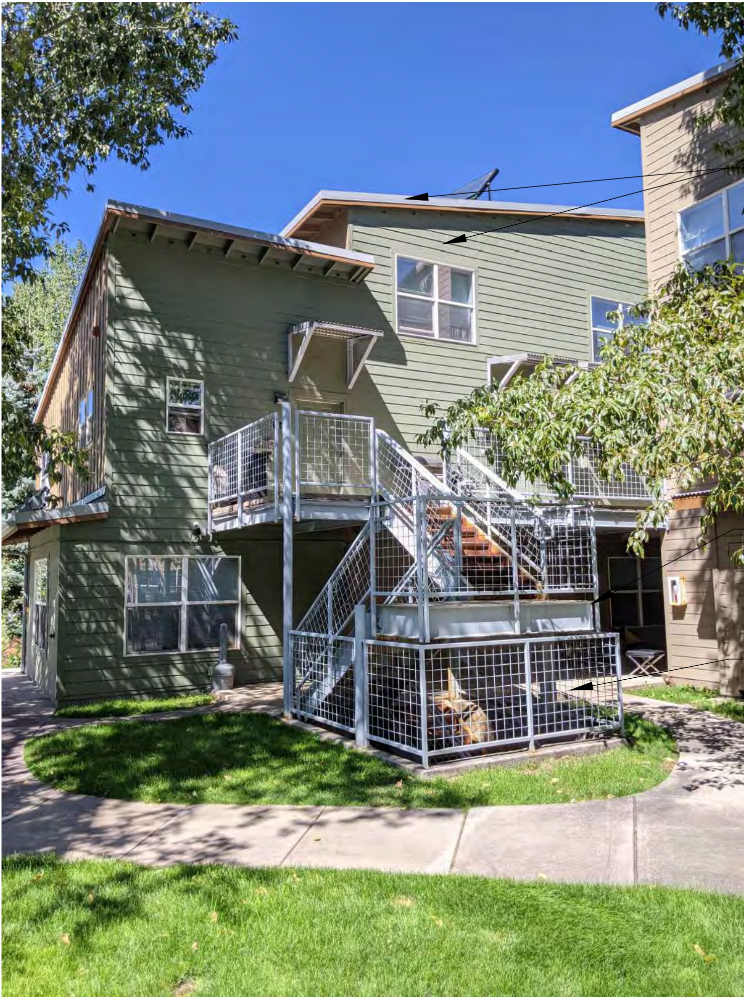
STAIR 10 (PHASE 1) EXISTING/DEMOLITION PHOTO 1 D1.4 NOT TO SCALE
