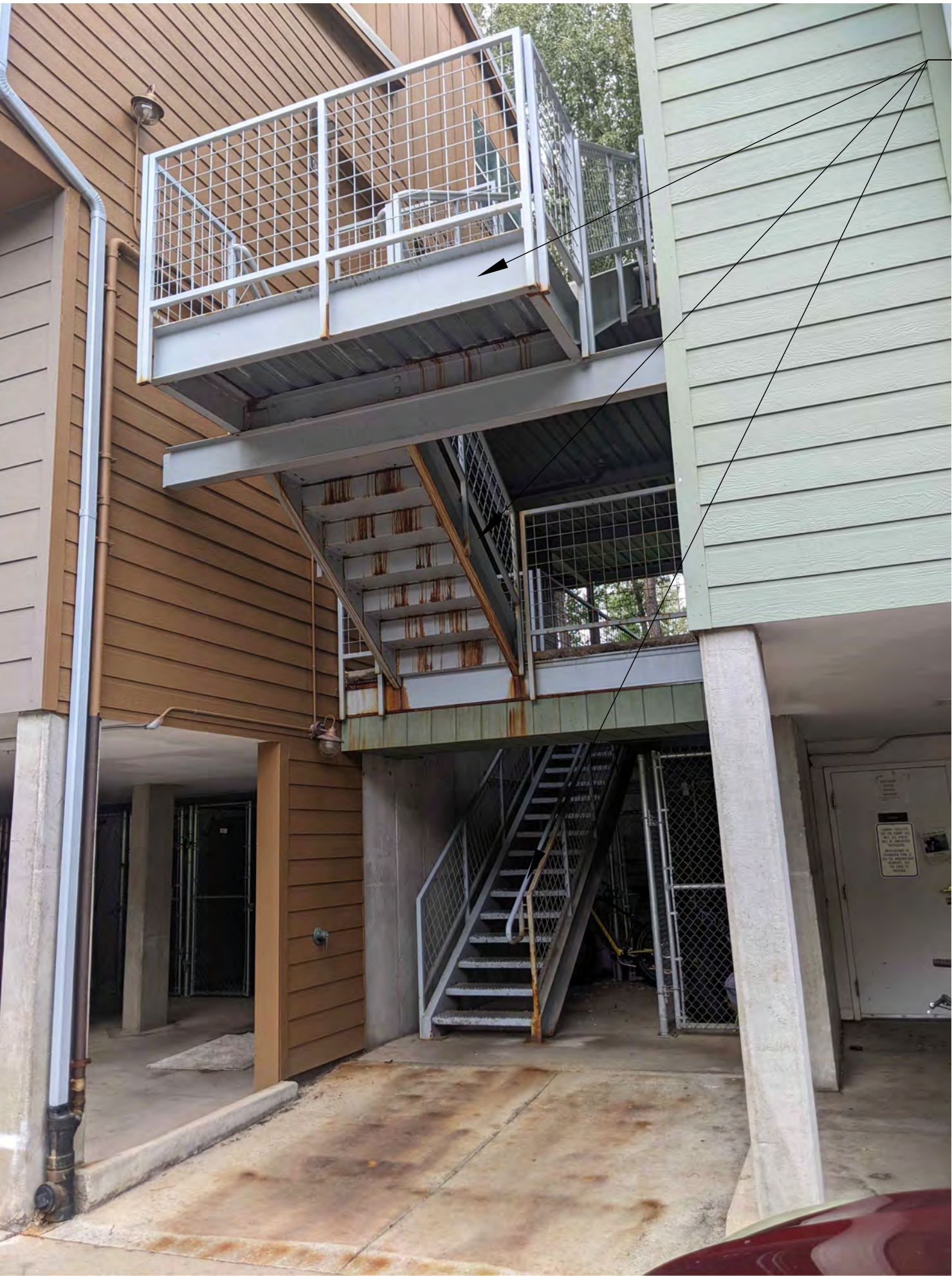
STAIR 900 (PHASE 5) EXISTING/DEMOLITION PHOTO 2 D1.4 NOT TO SCALE
