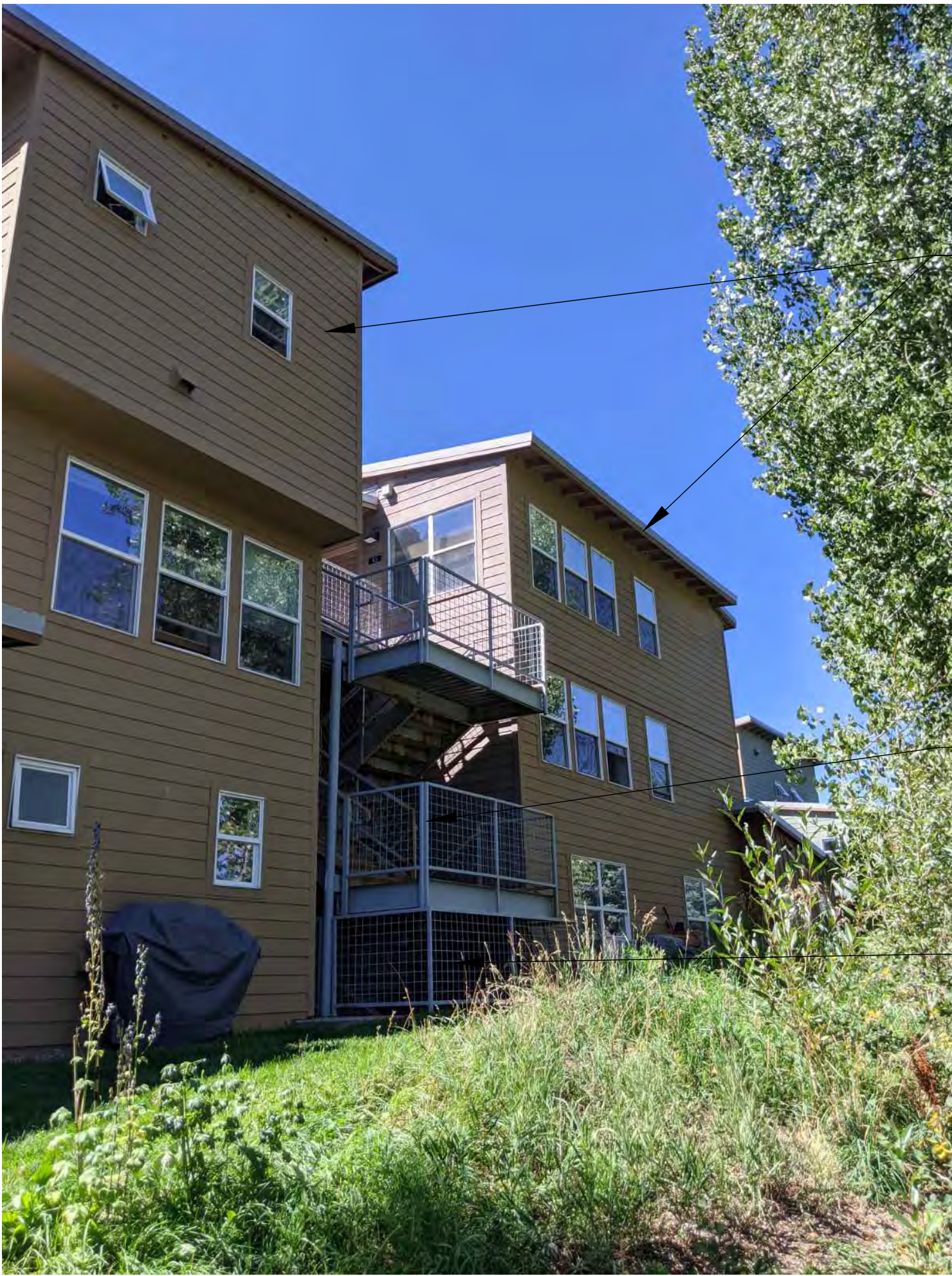
STAIR 40 (PHASE 3) EXISTING/DEMOLITION PHOTO 3 D1.4 NOT TO SCALE
