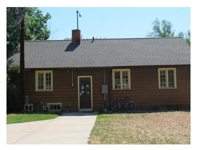
2. The Engineers Office Building is constructed primarily of wood, plaster, concrete and tarimpregnated composite roofing.
