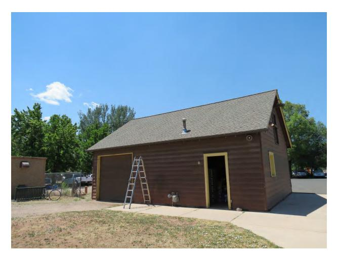
3. The Shop Building is constructed primarily of wood, drywall, concrete and tar-impregnated composite roofing.
